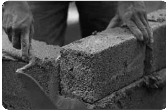
Grout was added to the walls to keep them strong.
